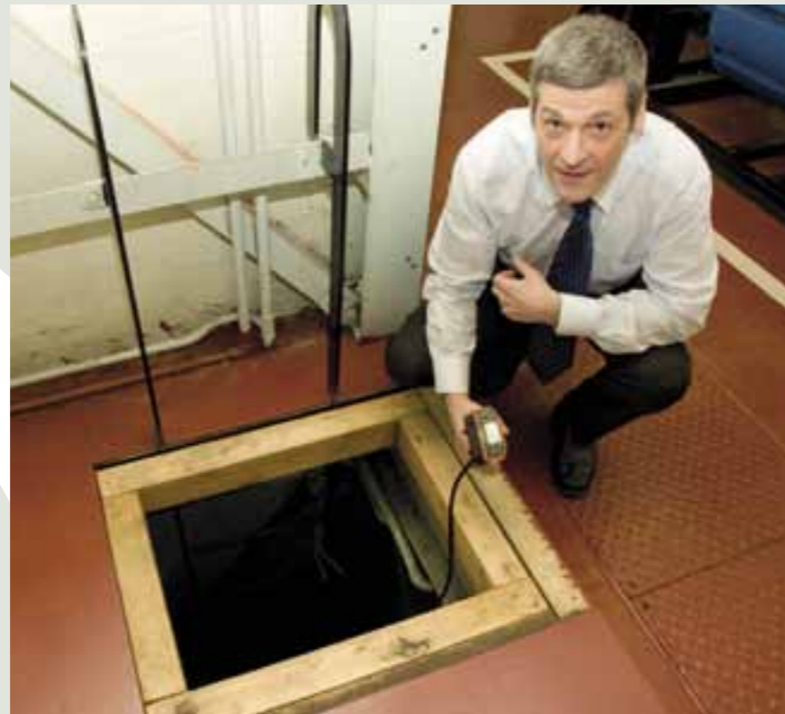
MEASURING OXYGEN LEVEL. Before entry the atmosphere should be tested to ensure that the normal oxygen level of 21% is present, says John Roach
